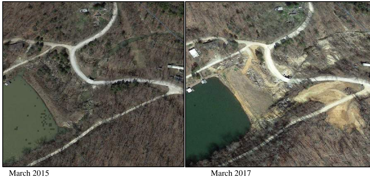
Figure 3.1.8- Glover’s Spring Lake Dam Failure
