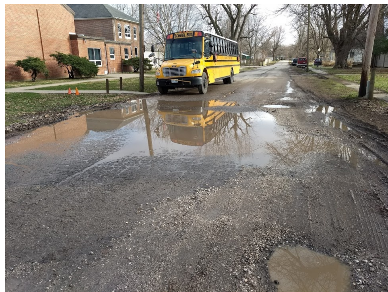
City of Blackwater awarded $304,050 in CDBG funding for road, stormwater, and ADA accessibility public infrastructure.
