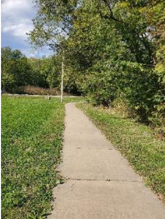
Good : Unlikely to hinder mobility of the average pedestrian. The sidewalk is free from significant cracking, buckling, gravel surfaces, or other debris which would impede pedestrian traffic.
