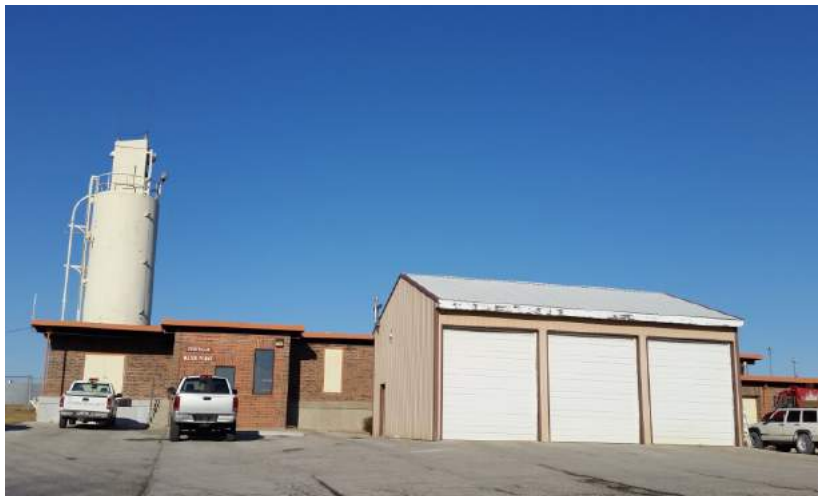
Figure 5.3 Centralia Water Treatment Facility on East Booth St.
