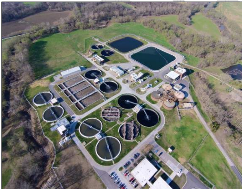
The Columbia Regional Wastewater Treatment Plant is a critical asset to effectively manage and treat wastewater from the City and surrounding area
