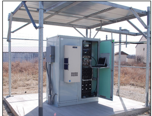
MOSWIN staff complete installation of base radios at a tower site.
