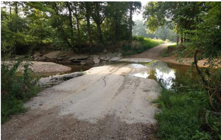
Moniteau County low water crossing.
