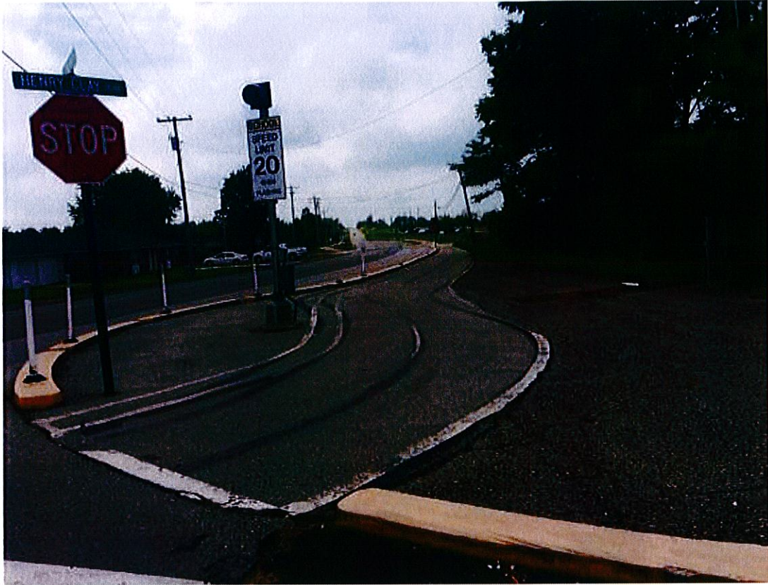
Main St. and Henry Clay Blvd. showing protected bike lane near South Boone Elementary School.
